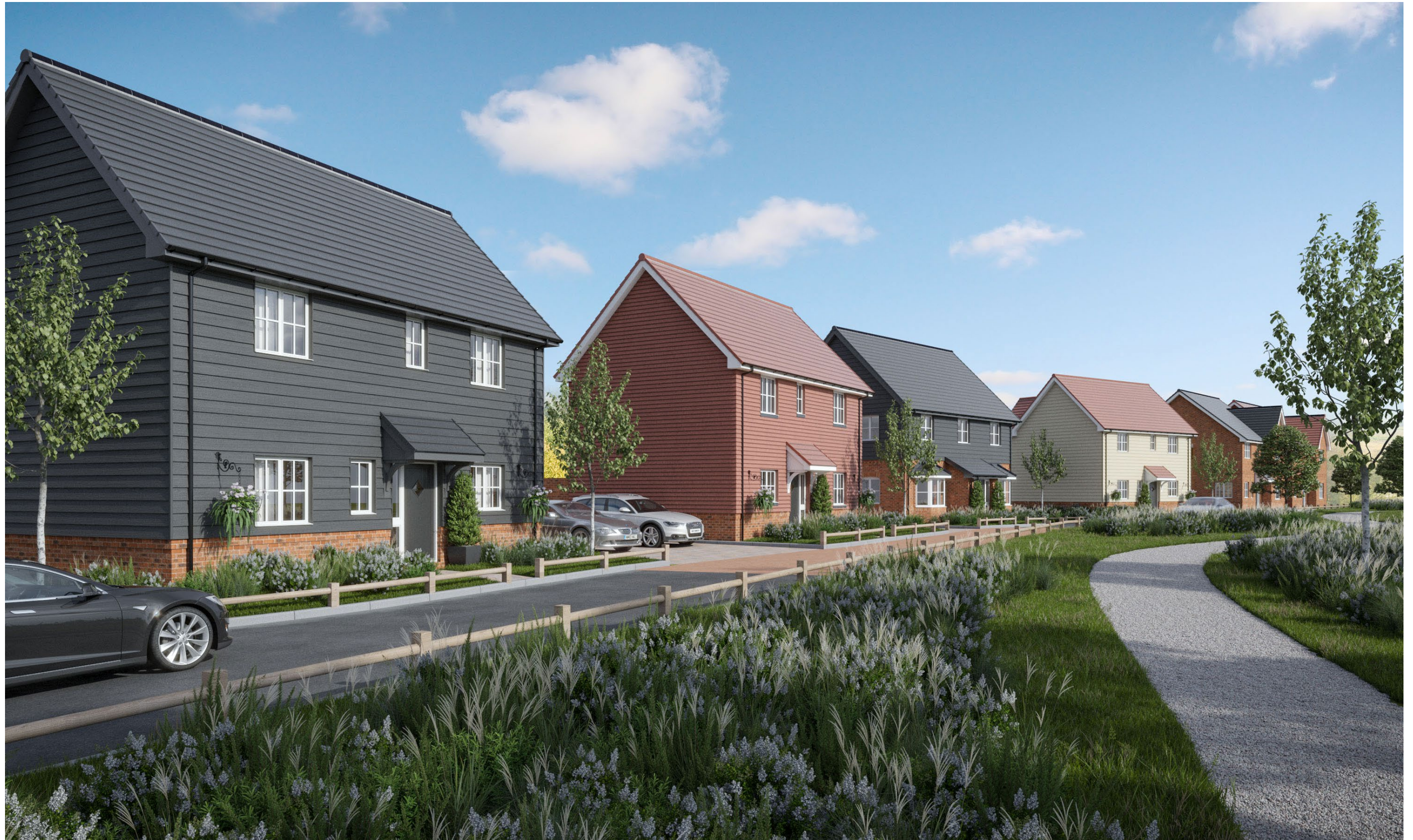
View North along Hillside Edge
